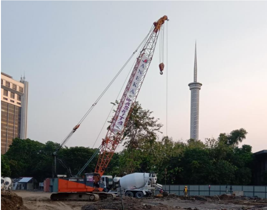
Istiqlal Mosque, Indonesia Foundation construction for new carpark development
