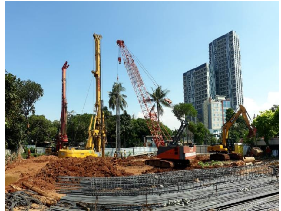
DAPENBI Project, Indonesia Foundation construction namely bored piling works
